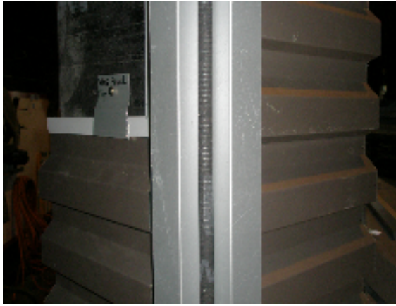
PICTURE PRIOR TO CAP INSTALLATION
