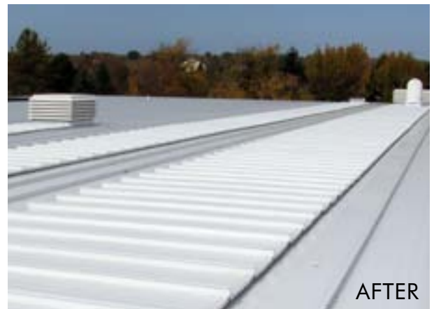
A completed retrofit utilizing Transverse Panel Curb detail.
